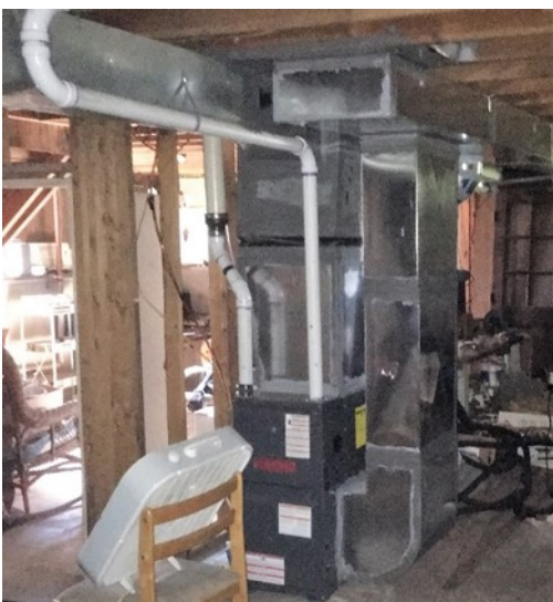
New Furnace and Duct Work
